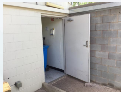
NO.: 2 PHOTO NO.: J154258-NT1009-PHOTO006 RESULT: ASBESTOS - PRESUMED NEGATIVE BUILDING/LEVEL: GHD BUILDING - GROUND LEVEL ROOM/LOCATION: LAB AREA - SOUTHWEST FEATURE/MATERIAL: FIRE DOOR - FIRE DOOR CORE SAMPLE NO.: SIMILAR TO: J154258-NT1009-002
