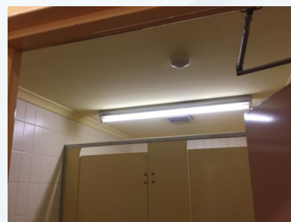
NO.: 6 PHOTO NO.: J154258-NT1009-PHOTO004 RESULT: ASBESTOS - NEGATIVE BUILDING/LEVEL: GHD BUILDING - GROUND LEVEL ROOM/LOCATION: TOILETS - THROUGHOUT FEATURE/MATERIAL: CEILING LINING - FIBRE CEMENT SHEETING SAMPLE NO.: J154258-NT1009-004
