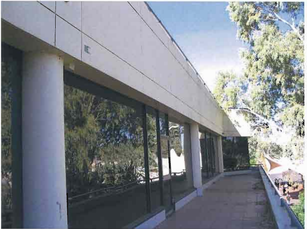
Photo No 5 External 1 st Floor – southern façade
