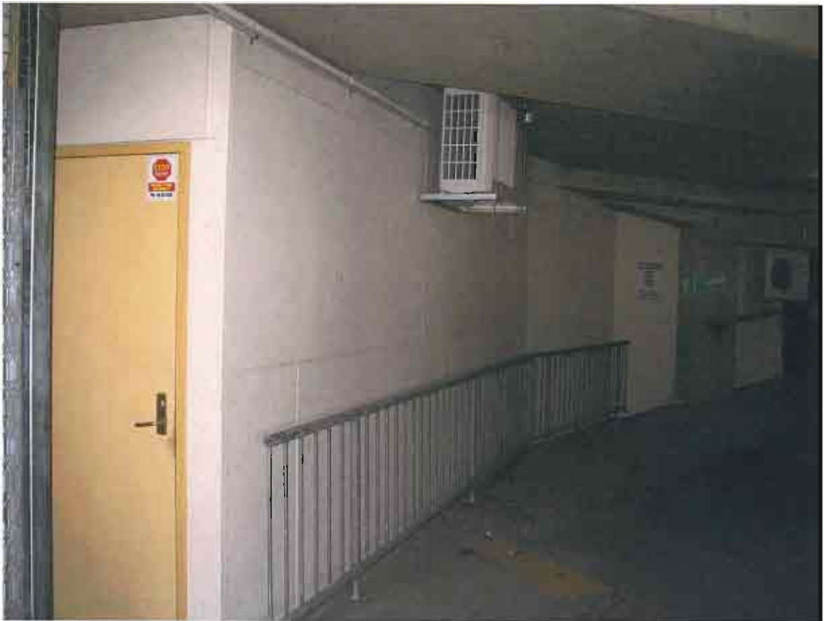
Photo No 11 Multi-Level Carpark northern wall (adjacent pub)
