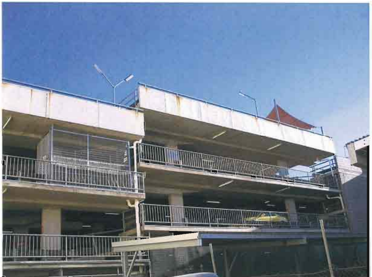
Photo No 12 Multi-Level Carpark northern side balustrade covering
