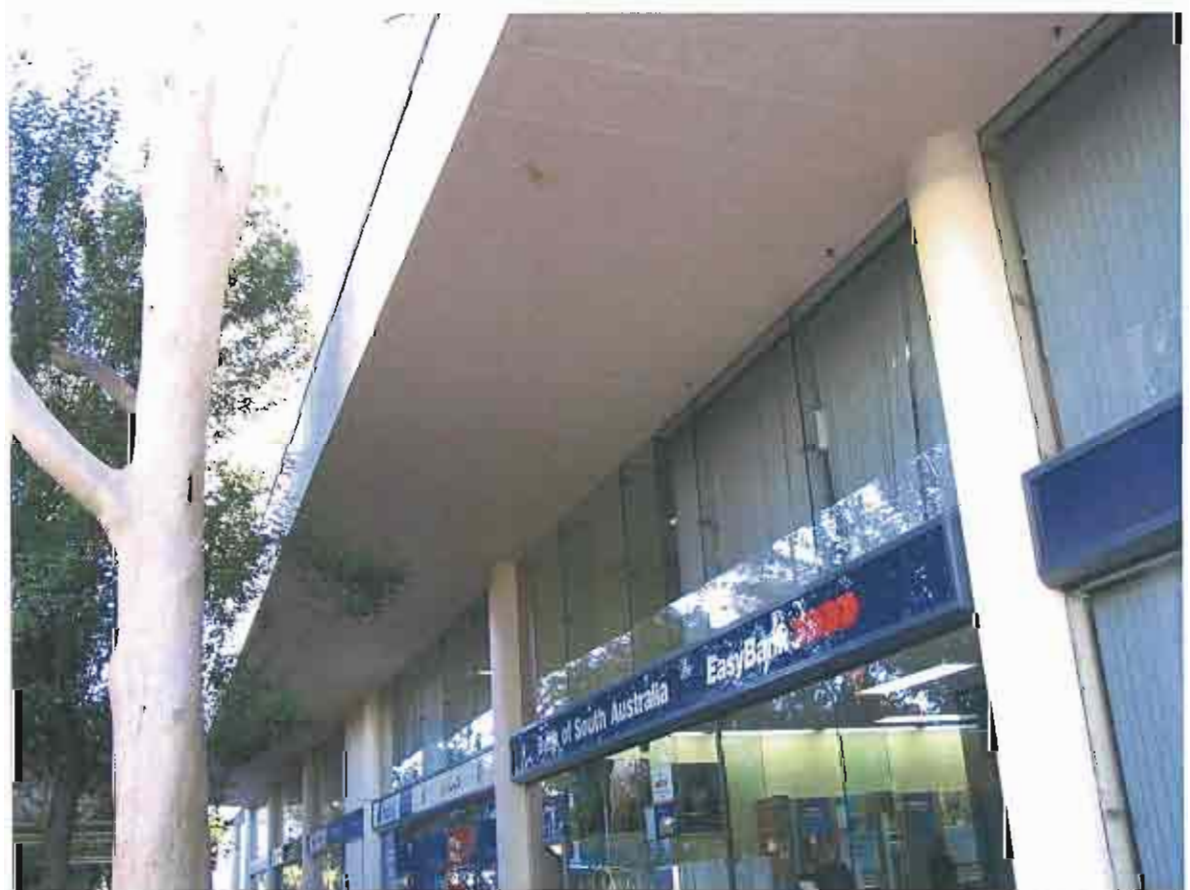
Photo No 4 Todd Street Mall – canopy ceiling lining
