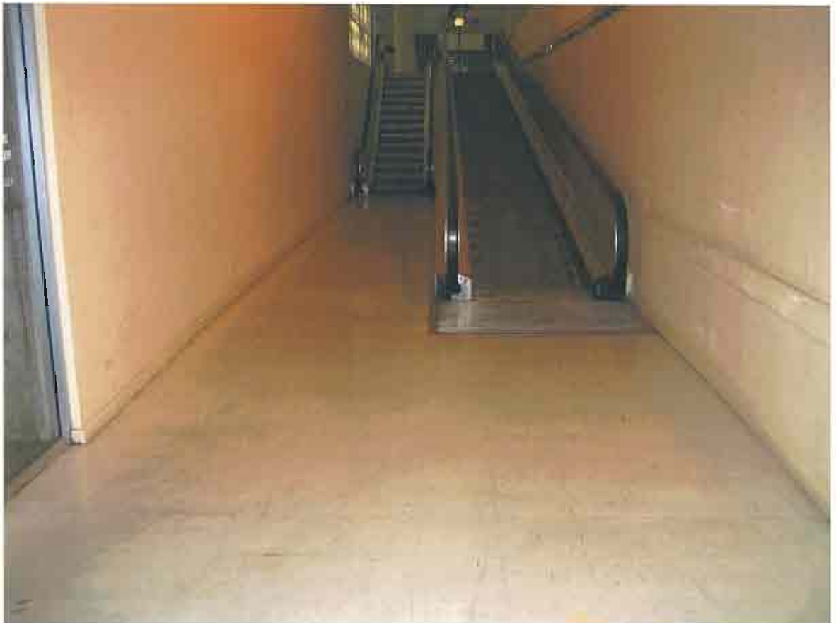
Photo No 24 Bi-Lo Carpark escalator foyer white vinyl floor tiles
