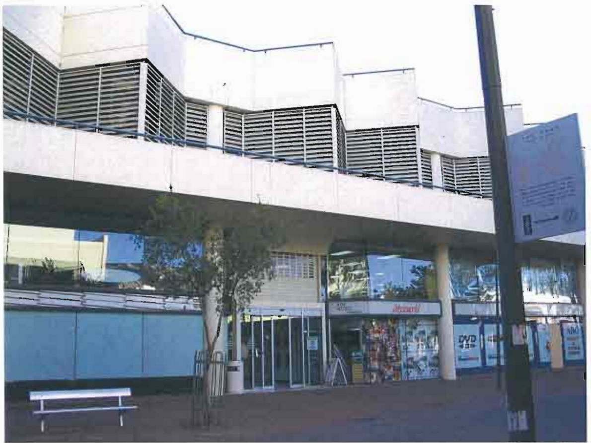
Photo No 3 Todd Street Mall - facade
