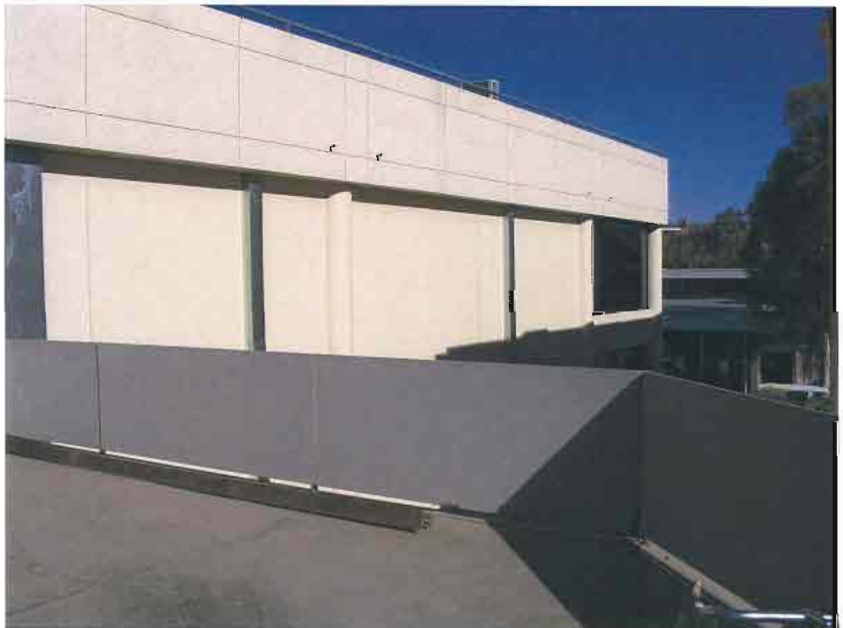
Photo No 6 External 1 st Floor – western façade and loading dock balustrade
