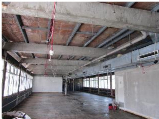
Asbestos cement ceiling tiles to the main building have been removed
