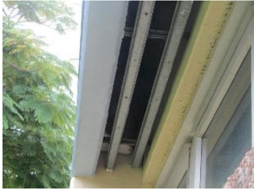
All asbestos cement roof eaves have been removed from the north facade of the annex building
