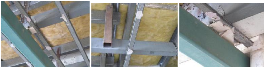
The walkway between the Main Building and the Annex had what appeared to be asbestos cement remnants adhered to soffit channels. These have all been removed. See next photos.
