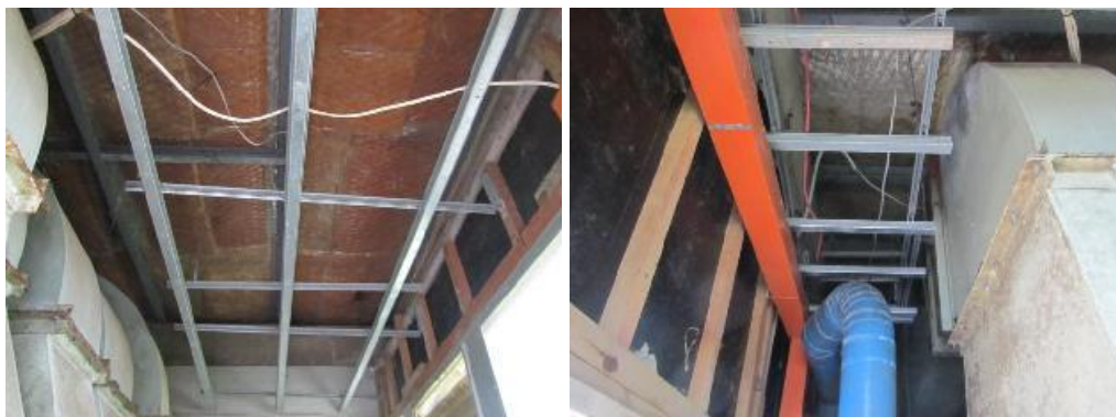
Asbestos cement linings to walls, ceilings and ducts in the plant room have all been removed.
