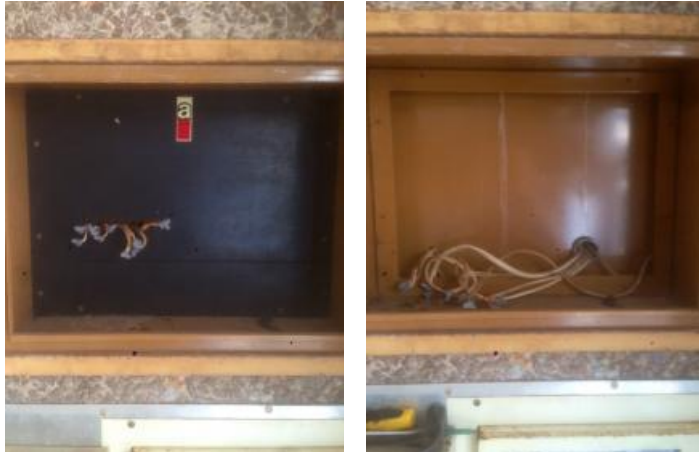
The asbestos containing electrical backing board located on the south façade of the Annex building has been removed.
