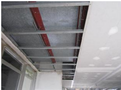
All asbestos cement roof eaves have been removed from the south facade of the annex building
