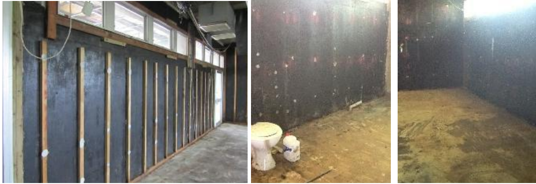
At the east end of the Annex building, battens containing asbestos cement fragments have now all been removed.
