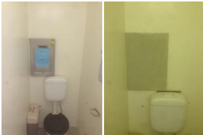
Sanitary disposal devices located in female toilets in the main building have all been removed.
