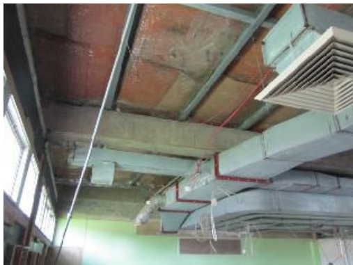
In the same space, all asbestos cement linings associated with the ceiling or ducting has now been removed.
