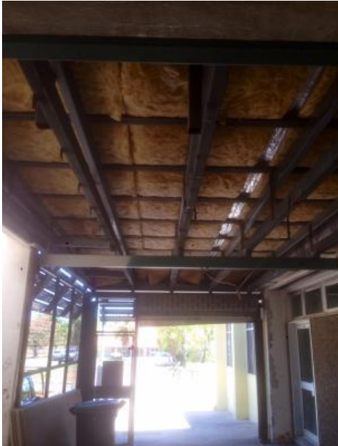
Photo shows furring channels to walkway removed.
