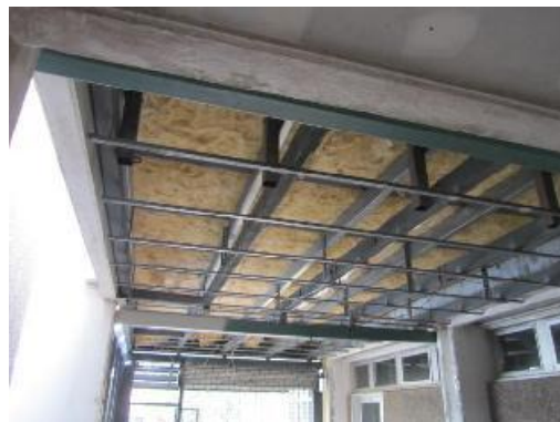
All asbestos cement soffit linings have been removed from the walkway between the main building and the annex building. Metal channels left in place and recorded as possibly having asbestos cement debris attached have been removed.
