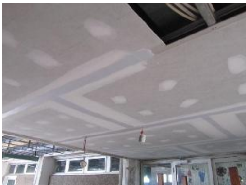
All asbestos cement soffit linings have been removed from the walkway between the main building and the annex building. Metal channels left in place and recorded as possibly having asbestos cement debris attached have been removed.
