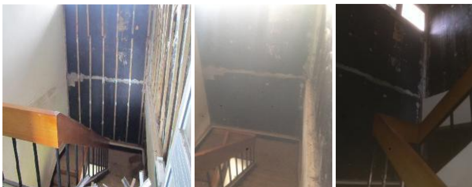
Battens containing asbestos cement fragments in stairwells have been removed.
