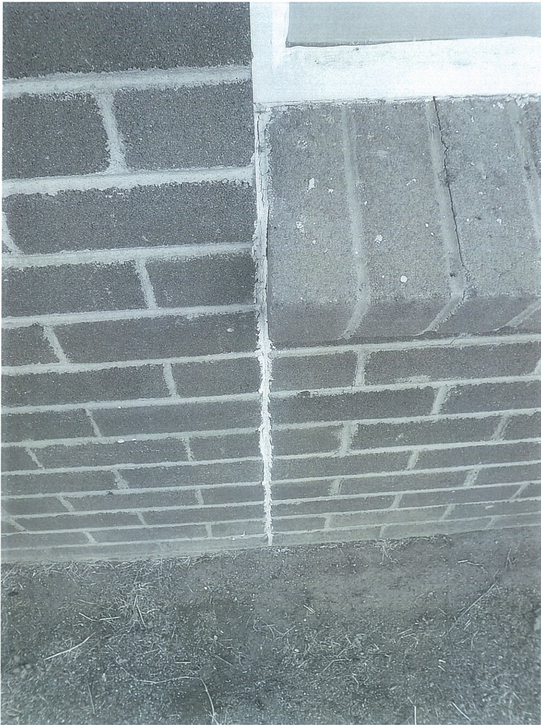
Building B- Expansion joint
