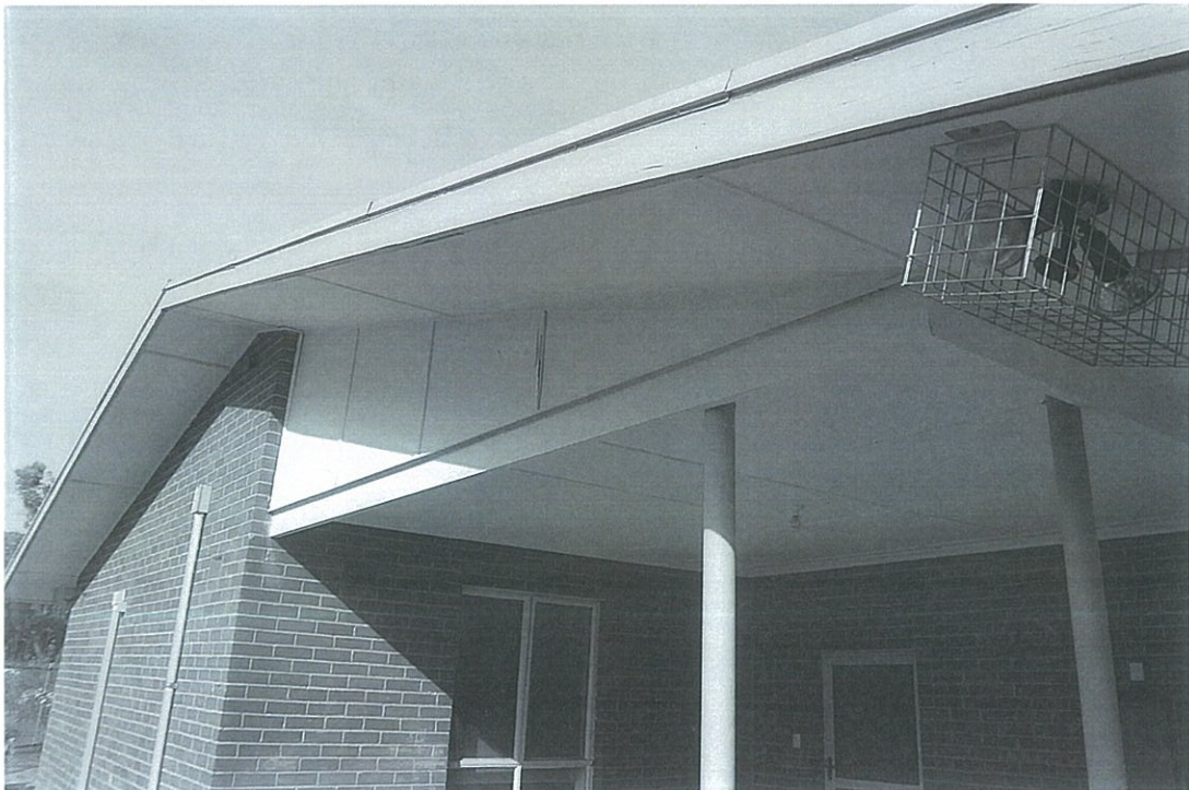
Building B- Eave lining and gable end.
