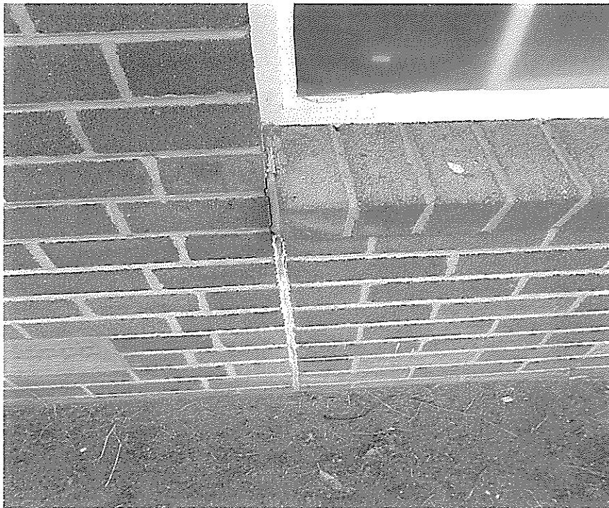
Building A- Joint sealant
