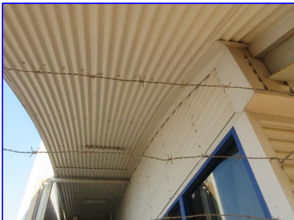
Photo 5 – External Eaves and Gables - Pressed Metal Clad to External of the Building
