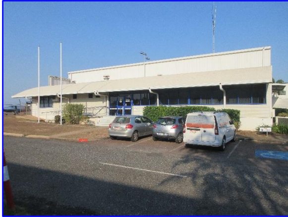
Photo 1 – Bristow Hangar, Lancaster Road, Eaton Looking West From Lancaster Road – Pressed Metal Clad and Blockwork to External of the Building
