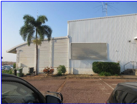
Photo 3 – Bristow Hangar, Lancaster Road, Eaton Looking From North to South, Administration Building on Left - Pressed Metal Clad and Blockwork to External of the Building
