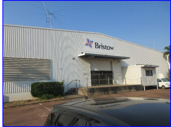
Photo 2 – Bristow Hangar, Lancaster Road, Eaton Looking From North to South - Pressed Metal Clad and Blockwork to External of the Building
