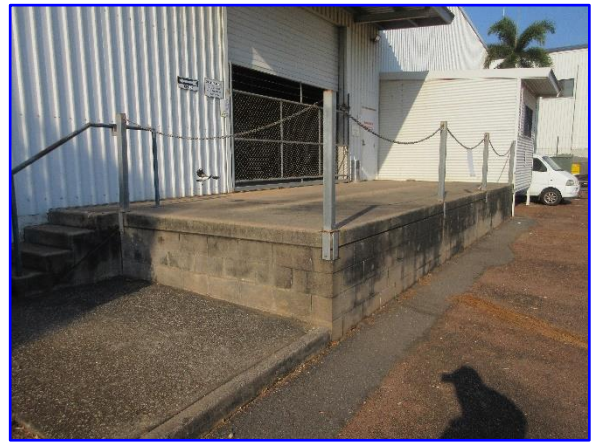
Photo 4 – Loading Dock and Add-On Building From Carpark - Pressed Metal Clad and Blockwork to External of the Building
