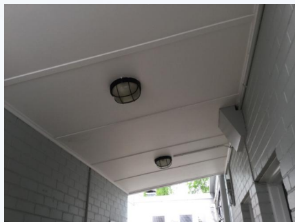
NO.: 2 PHOTO NO.: J159257-NT0557B-PHOTO007 RESULT: ASBESTOS - PREVIOUSLY SAMPLED POSITIVE BUILDING/LEVEL: NIGHTCLIFF LIBRARY - GROUND LEVEL ROOM/LOCATION: BREEZEWAY - THROUGHOUT FEATURE/MATERIAL: CEILING LINING - FIBRE CEMENT SHEETING SAMPLE NO.: PREVIOUSLY SAMPLED AEC 4-2013
