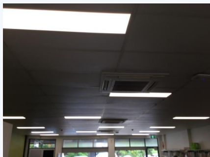
NO.: 3 PHOTO NO.: J159257-NT0557B-PHOTO008 RESULT: ASBESTOS - PREVIOUSLY SAMPLED POSITIVE BUILDING/LEVEL: NIGHTCLIFF LIBRARY - GROUND LEVEL ROOM/LOCATION: LIBRARY - EAST FEATURE/MATERIAL: CEILING LINING - FIBRE CEMENT SHEETING SAMPLE NO.: PREVIOUSLY SAMPLED AEC 1-2013
