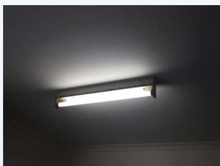
NO.: 4 PHOTO NO.: J159257-NT0557B-PHOTO004 RESULT: ASBESTOS - PREVIOUSLY SAMPLED POSITIVE BUILDING/LEVEL: NIGHTCLIFF LIBRARY - GROUND LEVEL ROOM/LOCATION: PUBLIC TOILET - THROUGHOUT FEATURE/MATERIAL: CEILING LINING - FIBRE CEMENT SHEETING SAMPLE NO.: PREVIOUSLY SAMPLED AEC AS PER 2-2013
